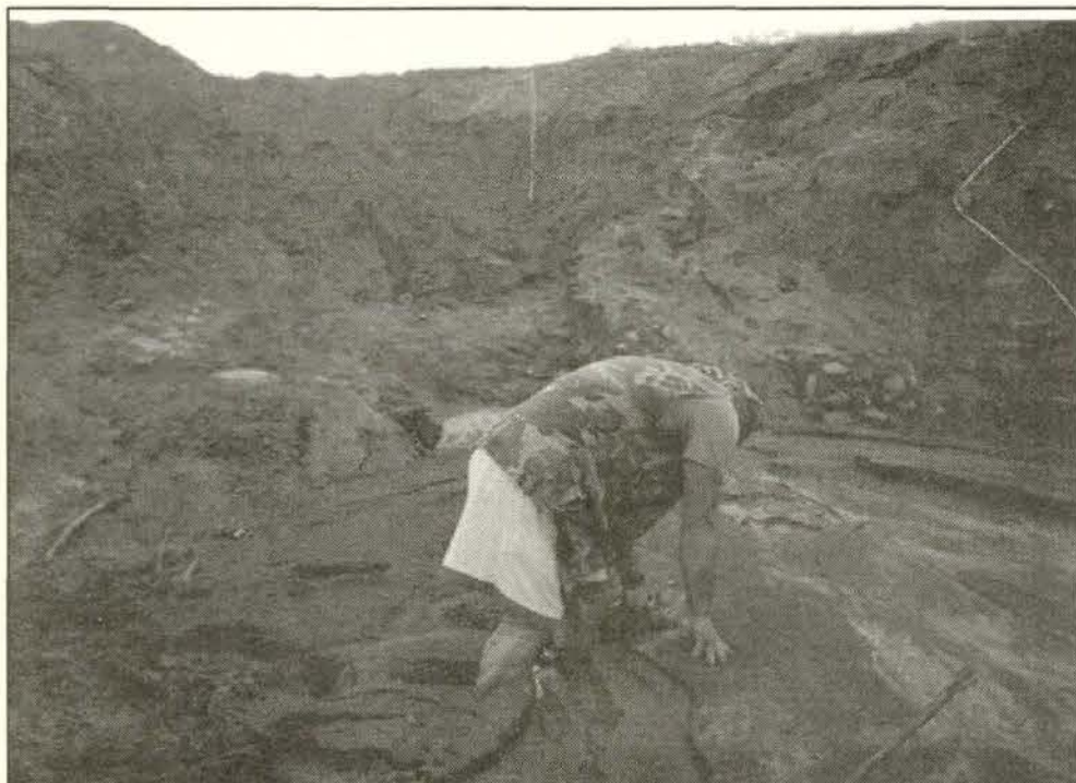
Winter rains caused heavy runoff in pipeline trenches.
