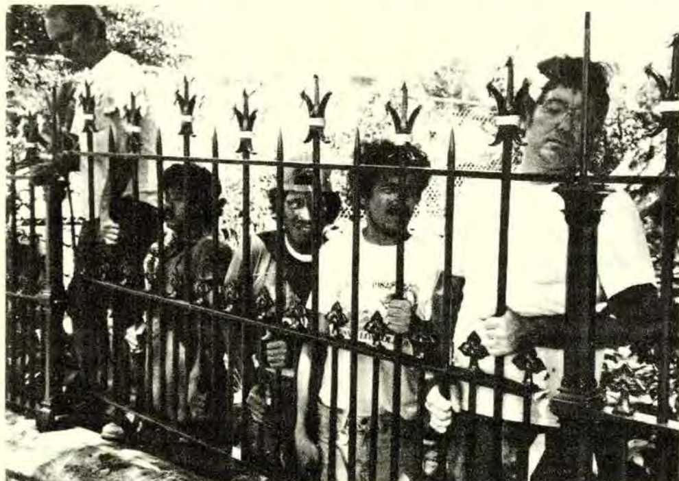
Workmen put section of fence in place after refinishing job. Note new placements on fence tips.
