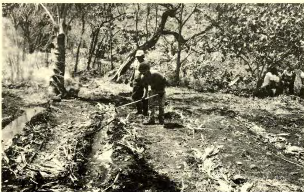
An irrigation ditch is being unclogged to let water flow freely.
